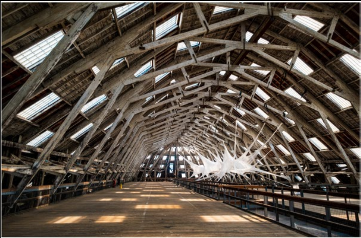
Covered Slipway - Chatham Dockyard ... (marc.barrot)
